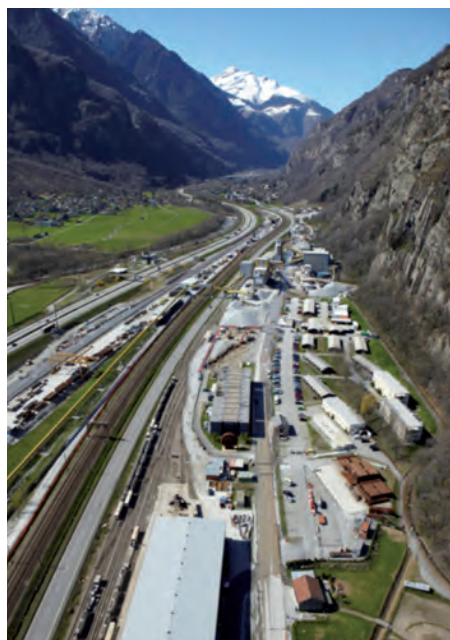
Figure 18 : Rig area of a major tunnel project - the heart of logistics® ATG
