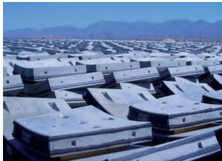
Figure 8 :Stored precast concrete segments ready for supply to the tunnelling work for a water supply project. The logistics and supply of this type of tunnel support are extensive and needs to be considered early in the tunnel planning phases. © Daetwyler
