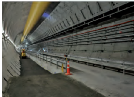
Figure 3 : Top right: Pipe-jacking tunnel as water sewer Lower right: Backfilling the gaps aside of an invert gallery in a large tunnel parallel to tunnel excavation © Babendererde Engineers
