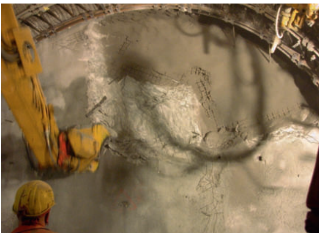
► Figs 15a and b Excavation and immediate sealing of the face (left); installation of the face bolts using the Jumbo Axera T12 (right)
