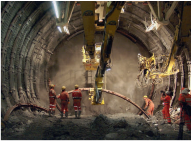
► Figs 16a and b The rock support installation equipment in use (left); cutting of the face bolts to length (right)
