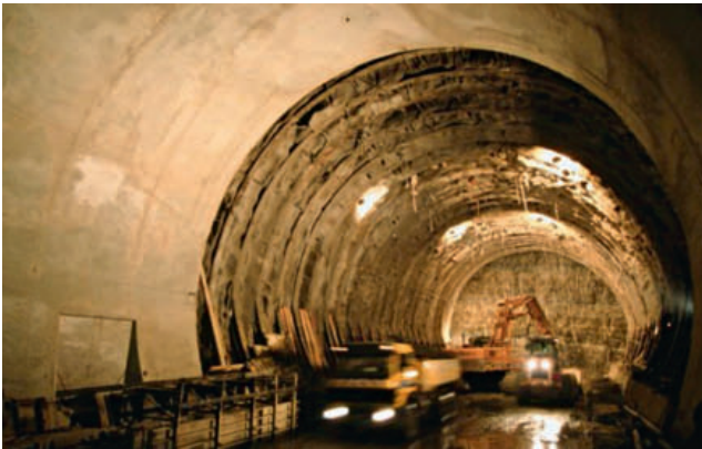
► Fig. 6 Example of tunnelling on the resistance principle
