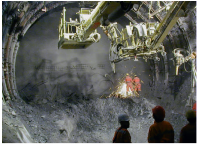
► Figs 16a and b The rock support installation equipment in use (left); cutting of the face bolts to length (right)
