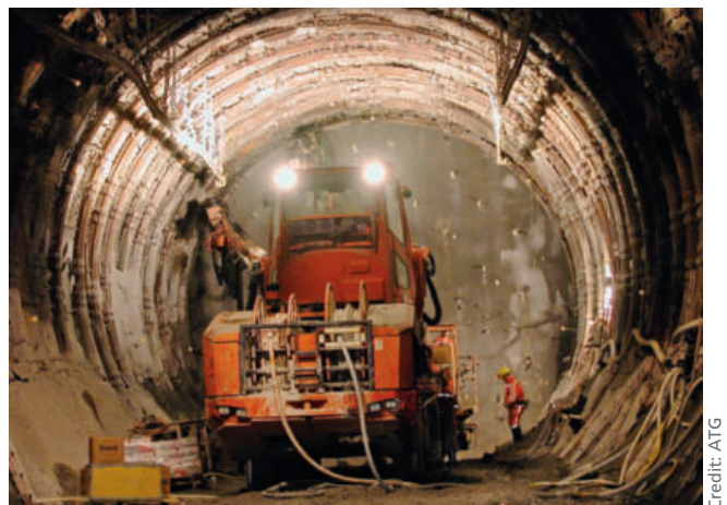
► Figs 15a and b Excavation and immediate sealing of the face (left); installation of the face bolts using the Jumbo Axera T12 (right)
