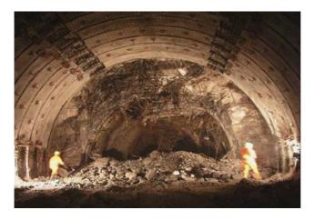
Figure 13: Tunnel reconstruction in the multifunctional station Faido due to heavy squeezing
