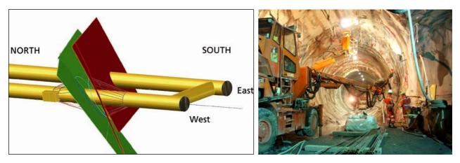
Figure 10: Grouting of a fault zone
