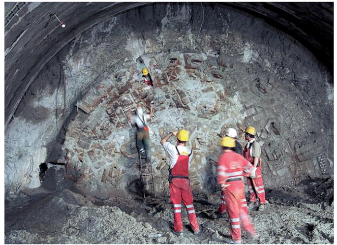
Fig. 8. Cutterhead of Amsteg West TBM exposed (15 November 2005)
