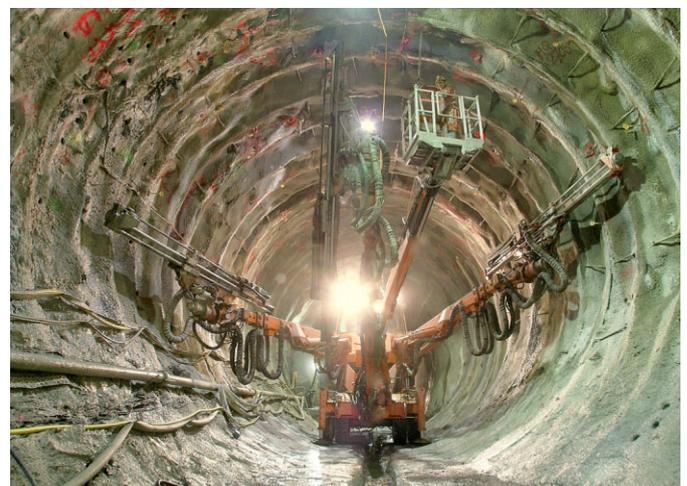
Fig. 11. Drilling grouting holes with tunnel jumbo
