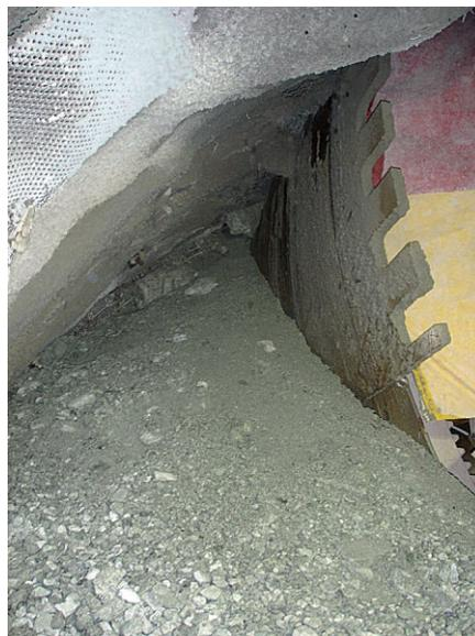
Fig. 3. Amsteg West: side niche next to cutterhead filled with stone inflow
