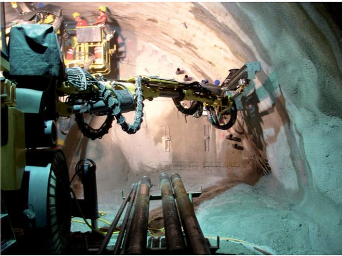
Fig. 7. Opposite drive at Amsteg West, installation of pipe screen
